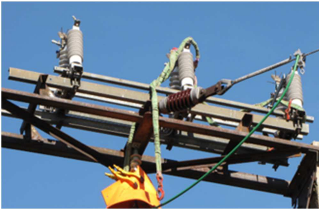
Fig. 3. The pole-mounted switch partially prepared for lifting.
