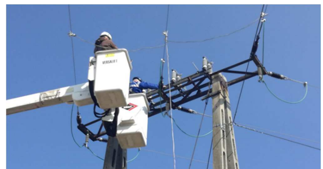
Fig. 6. Accident reconstruction on the pole.
